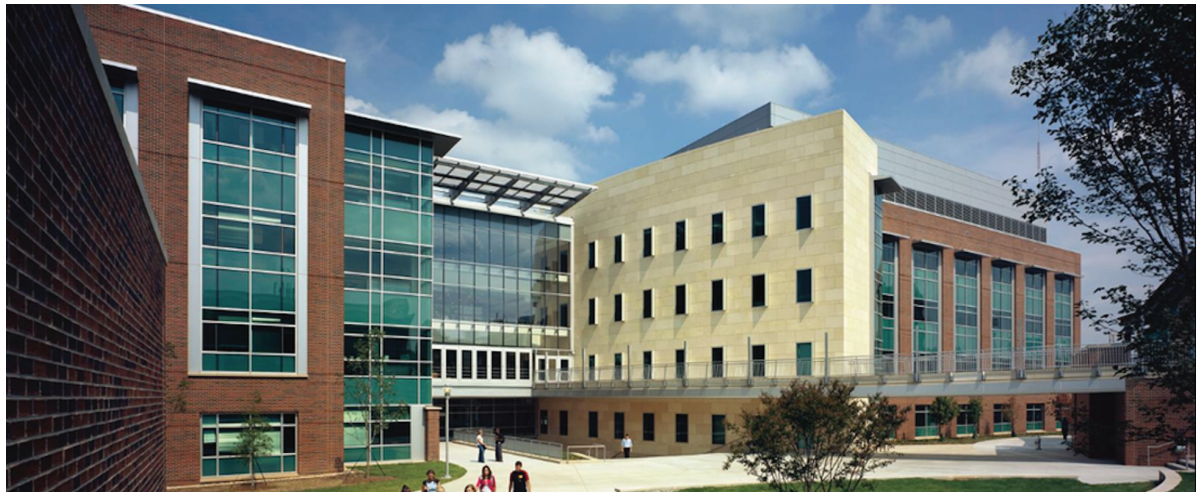
The REVEALS project is headquartered in the Molecular Science and Engineering Building on the main campus of the Georgia Institute of Technology in Atlanta, Georgia. Additional facilities are located at the partner institutions.
